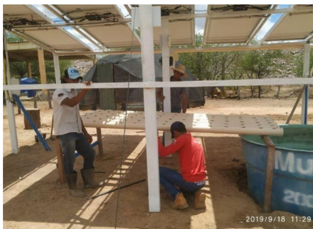
Figure 37 - Agrivoltaic system and assembly of aquaponics system below the modules
