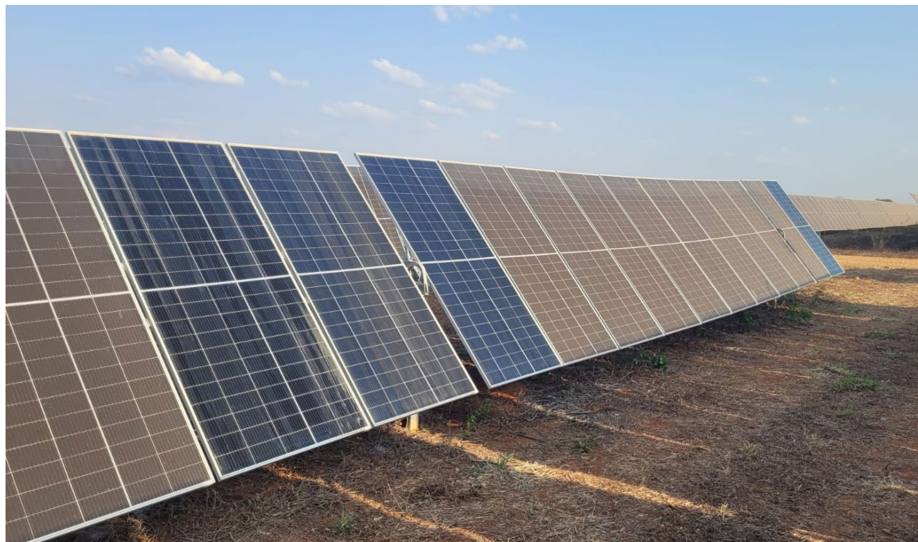
Figure 60 - Example of dirty modules and clean modules
