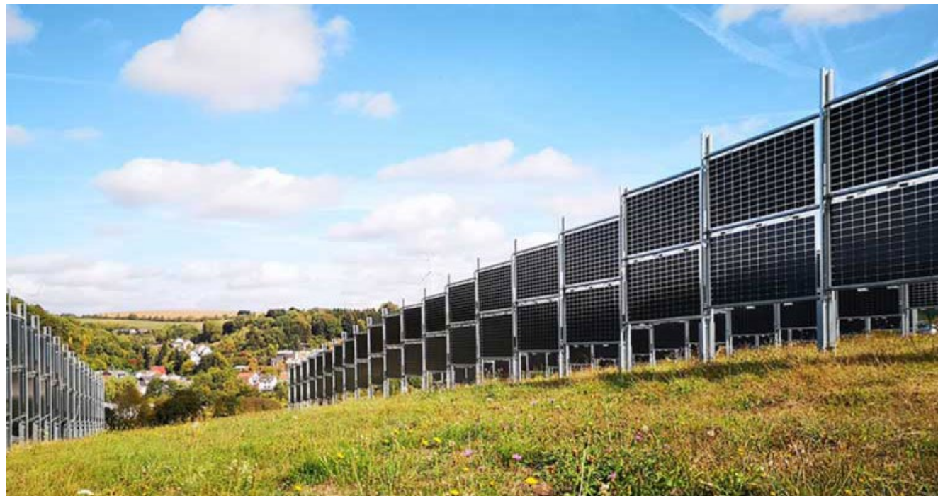
Figure 62 - Bifacial, vertically installed PV modules for fencing applications
